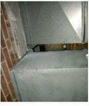
After another call to our heating contractor, the duct was reattached and ready for the suspended ceiling repair.
