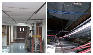
I quickly called a a company that specialized in the installation of suspended ceilings to come out and wire up the ceiling so it won't collapse any further. When the technician arrived and started to wire up the ceiling he noticed that the large heating duct that connects the Bear Room to the Augsburg Alley classrooms had pulled
