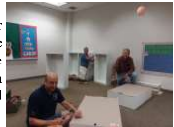
Assembly & Installation of Bookshelves in New Children's Library
