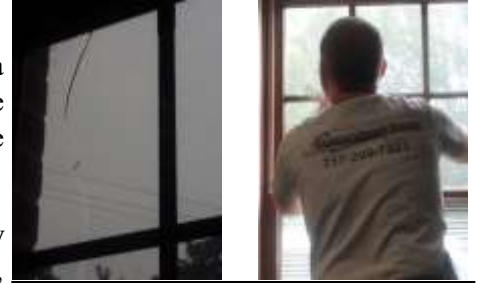
Augsburg Window Repair
