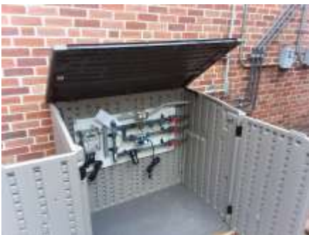
New Chemical Control Panel for Cooling Tower in Old Section
