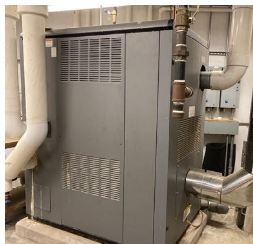
Rebuilt Boiler (Sanctuary) & Installed Control System
