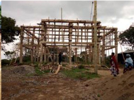
Walls being erected in August 2020
