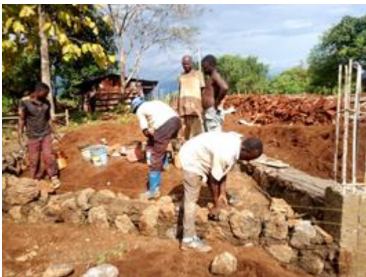
Laying foundation stones in March 2020
